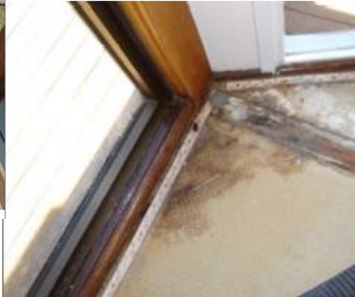
Water affected floors due to leaking windows
