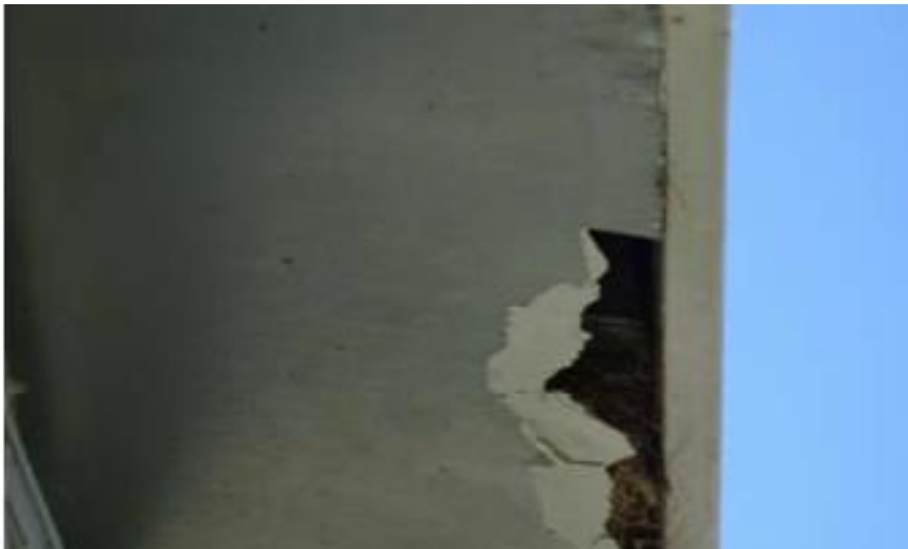
Significant damage to eaves
